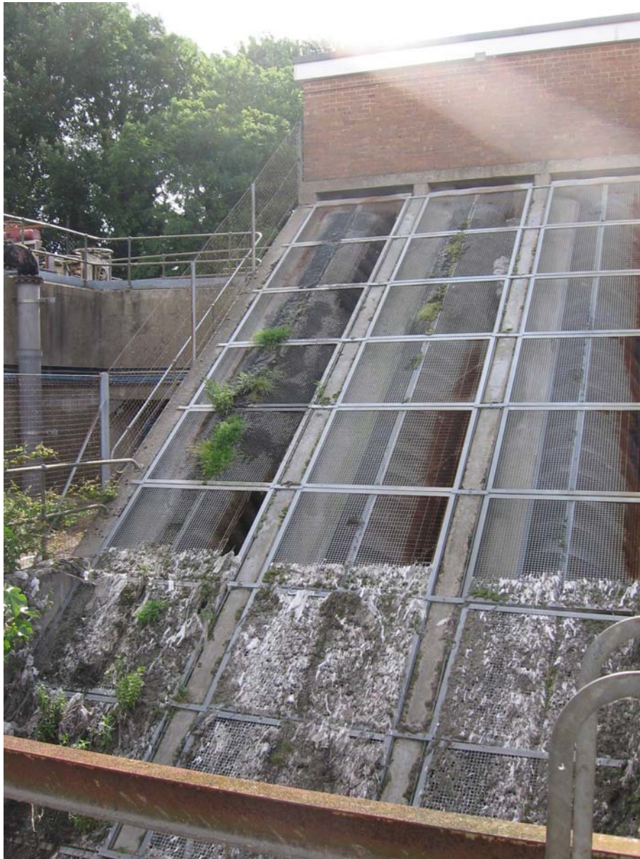
Figure 1 Inlet well and 3 archmides screws
