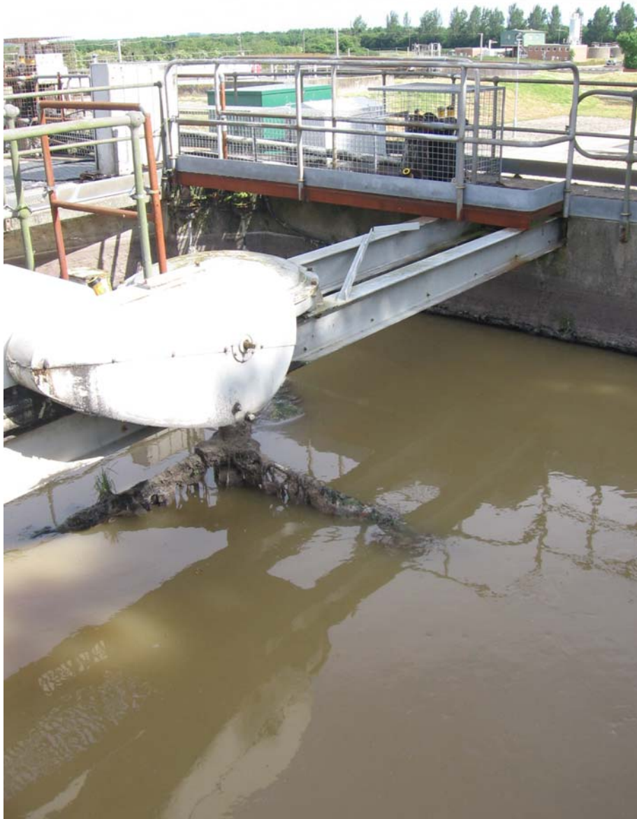
Figure 2 Grit settling tank
